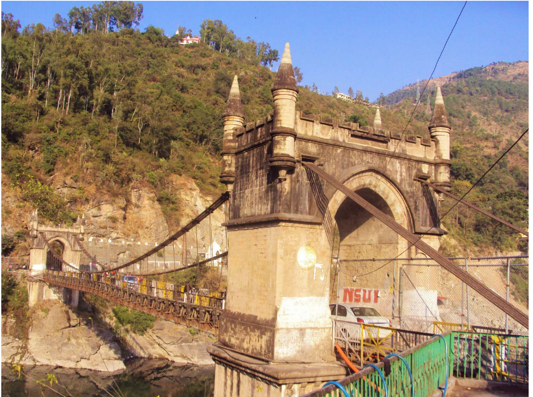
Another view of Victoria Bridge
